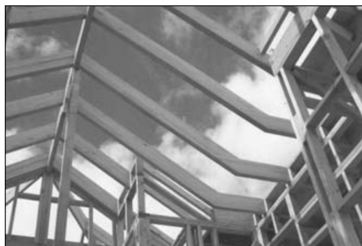
The clean lines and cranked shape of these pitched Glulam rafters illustrate the versatile roof forms possible using laminated timber.
