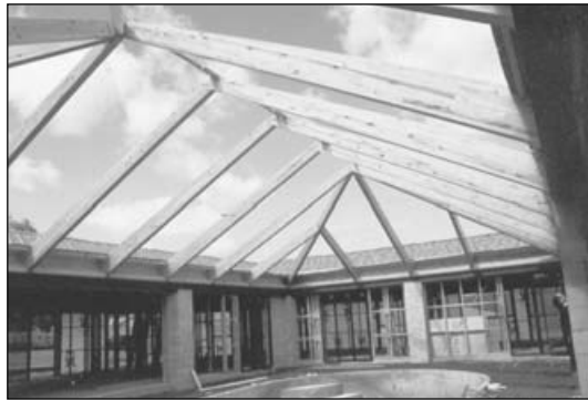
The solution for large open spaces is found in the strength and simplicity of Glulam roof frames.
