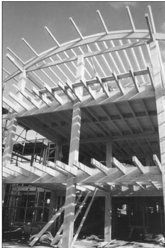
Three-story post and beam structure creates a unique feature demonstrating timber's natural strength and design possibilities.
