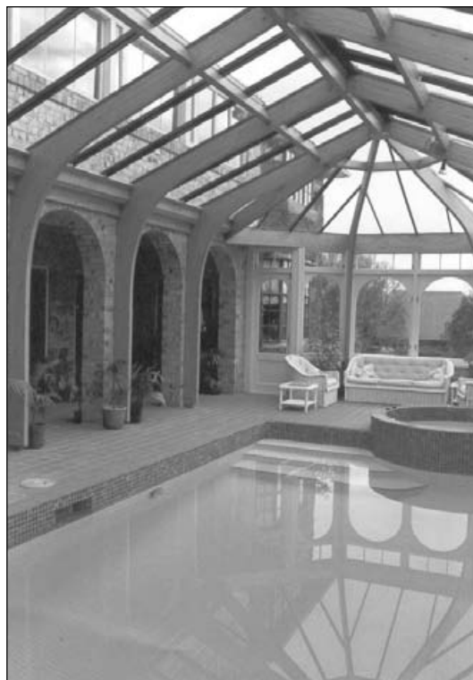
Curved Glulam portals highlight the design flexibility and natural beauty timber can bring in an indoor – outdoor situation.
